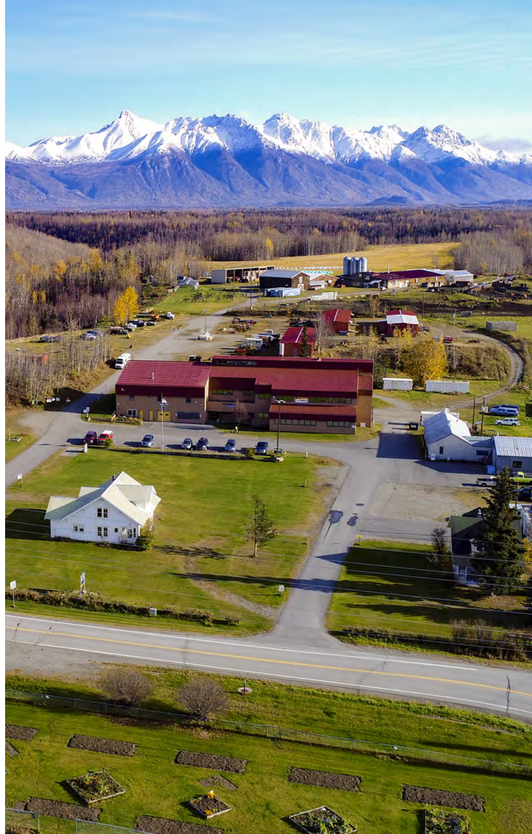
MEFEC Core Facilities Area with the Chugach Mountains in the background.
