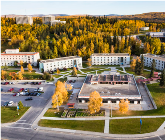
The four lower dorms are planned for demolition. Photo by JR Ancheta.
