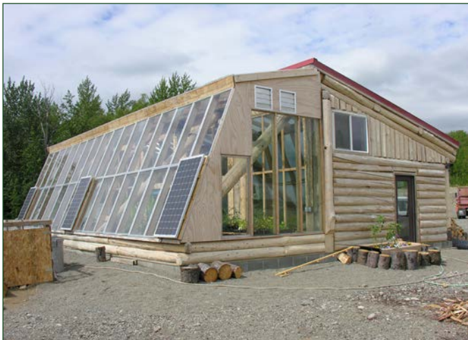
A slant-leg greenhouse in Chickaloon Native Village. Glass is used for the south wall.
