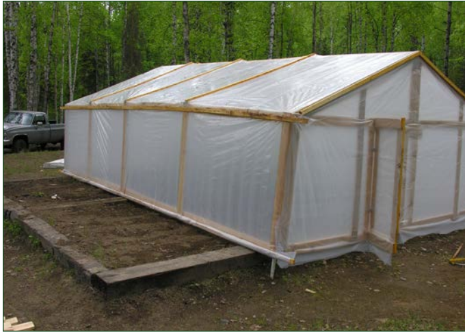
Plastic film is the least expensive type of greenhouse covering, but a greenhouse-grade plastic will only last 4-10 years.
