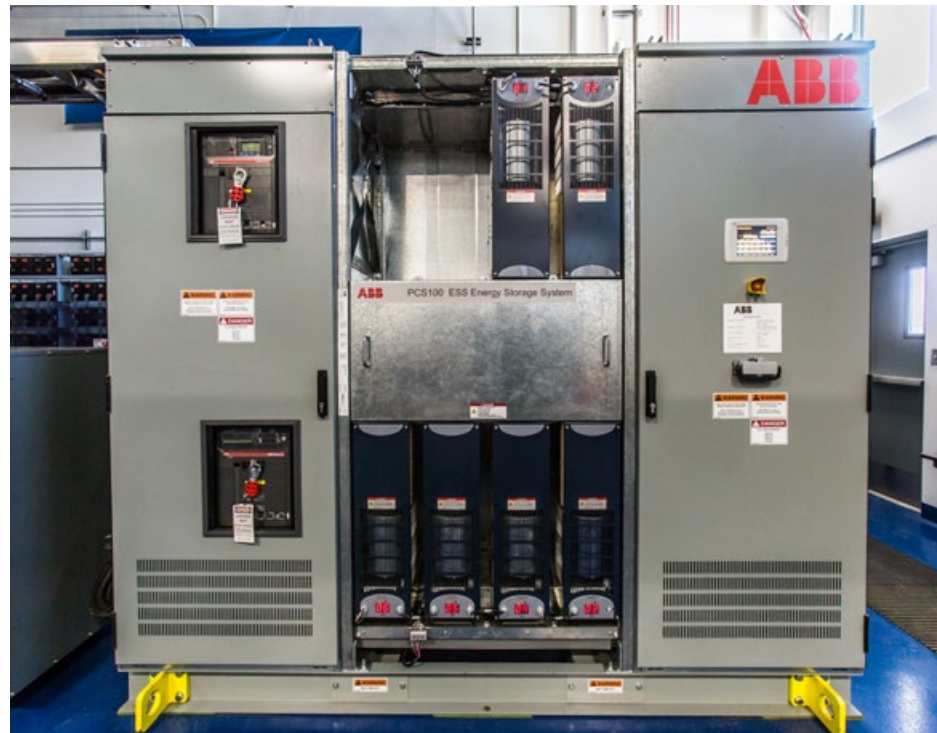
Above: A new ABB Inverter was purchased by ACEP for the testing of Hatch's flywheel system. UAF PHOTO BY TODD PARIS
