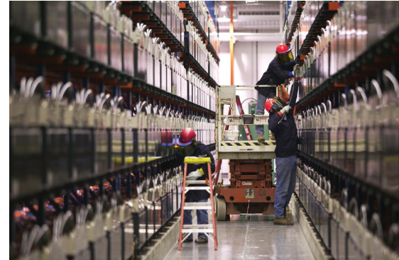
The 27 MW battery energy storage system (BESS) is one of Golden Valley Electric Association's initiatives to improve the reliability of service to residents of Fairbanks, Alaska.
