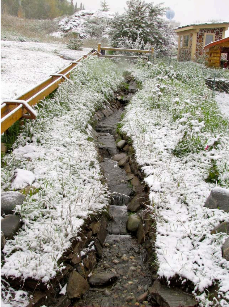
Recently repaired stream section covered with new sod.
