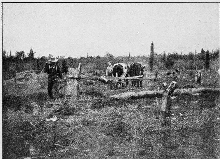
FIG. 2.—STUMP-PULLING TACKLE.
