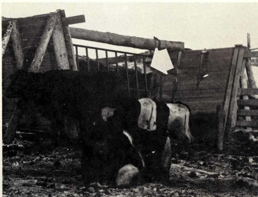
Arrow points to snow accumulation on top of silage, caused by settling after filling below top of walls. Filling to greater depth helps shed snow. Concrete floor and feeding apron eliminates soggy footing.
