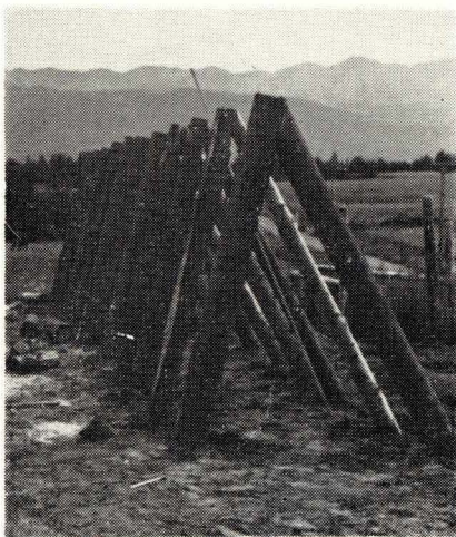
Close-up of post, brace and side-wall details.
