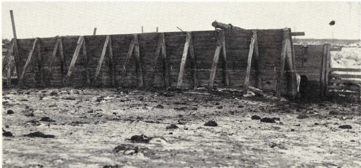
A simple drive-through bunker silo built of treated posts and rough-cut lumber. Materials cost estimate for this 100-ton storage is estimated at less than $500.
