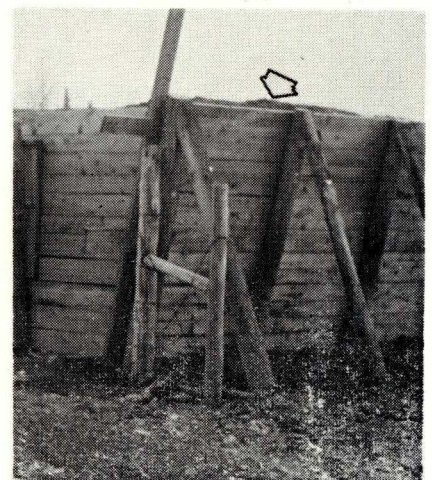
Arrow shows top of silage above top of wall. Filling above walls keeps snow from collecting on top.
