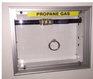
Figure 2. Propane gas shut-off valve
