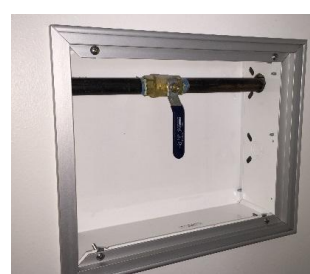
Figure 4. Valve handle in "off" position
