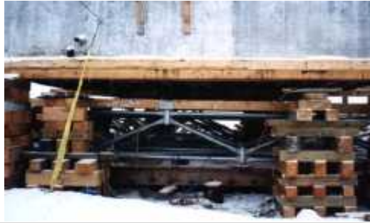
Photo 1: House on Cribs as Triodetic Frame is Installed.
