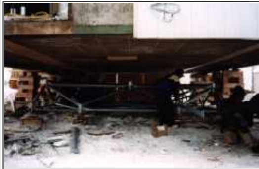
Photo 6: Assembling the Triodetic Space Frame Underneath a Crib Supported House.
