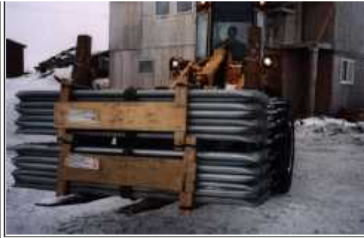
Photo 5: Unpacking the Tubular Triodetic Space Frame.
