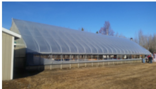
Greenhouse in Interior Alaska. Side curtains can be opened to allow for ventilation and cooling during the warmest months of the growing season.
