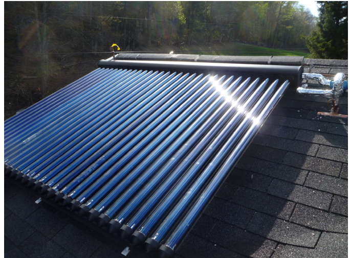
Figure 2. An evacuated glass tube with heat pipe.
