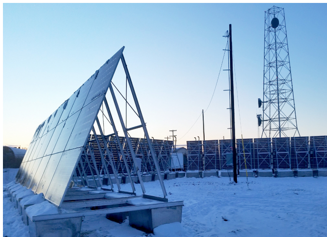
The solar PV array in Noorvik uses bifacial panels and has multiple orientations. Photo courtesy Rob Bensin
