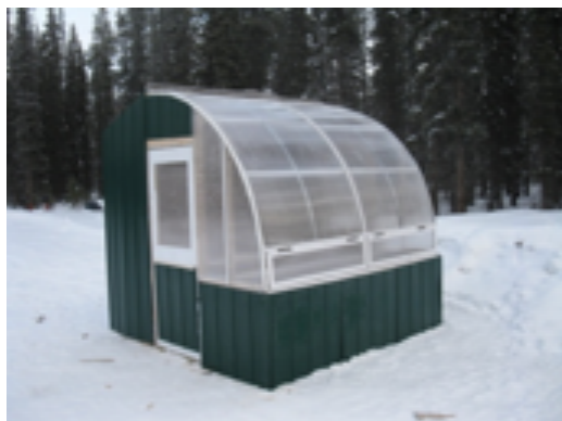
Three-season greenhouse. The north-facing wall is fully insulated. The sun's heat is stored in rock beds. A small circulation fan powered by a small solar panel forces air through PVC embedded in the rocks.
