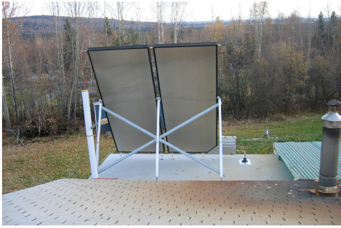
This photo from the rear of the collectors gives some idea of the tree shading to the south.
