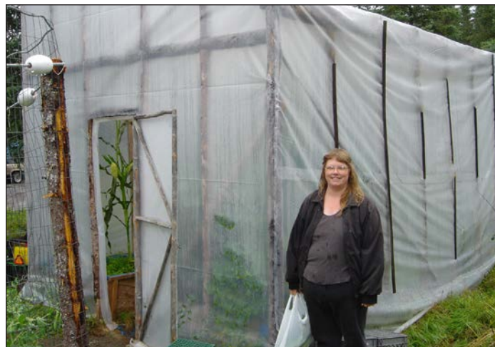
Picture 1. Door vents and high ceilings in small greenhouses can provide adequate ventilation.
