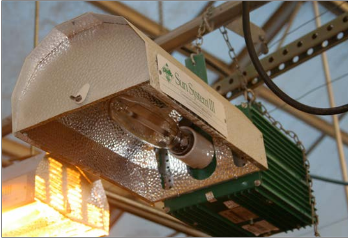
Picture 6. HID lamp with bulb, reflector and ballast/capacitor
