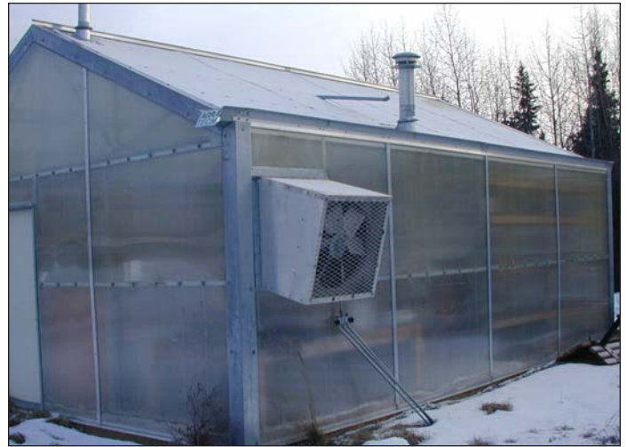
Picture 4. Freestanding greenhouses usually have fans at one end of the house and vents on the other.
