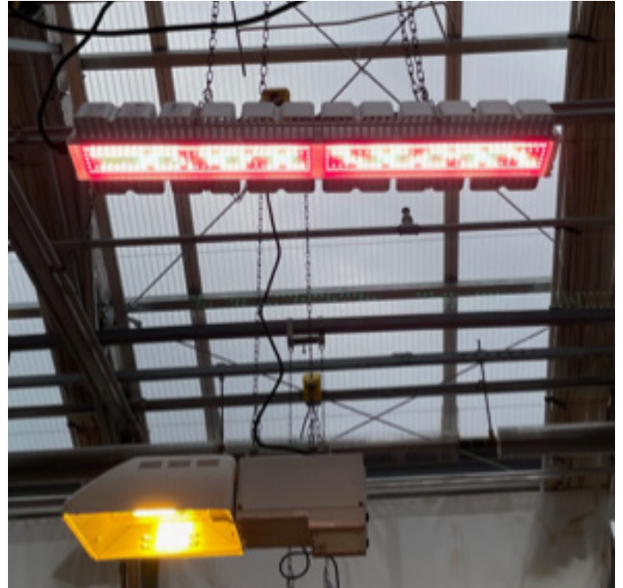
Picture 7. Greenhouse overhead LED fixture. For comparison, the light source at the bottom is the currently often used high pressure sodium (HPS) fixture.
