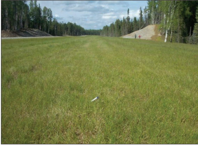
Figure 3. The Arctared red fescue grass planted on this runway has the potential to greatly reduce damage caused by rocks. The grass also reduces dust. Photo by Jud Scott
