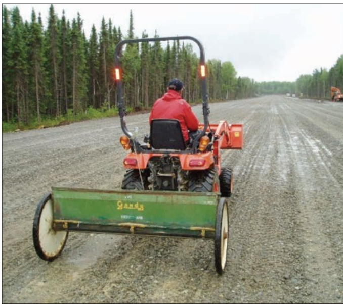
Figure 5. A tractor with a drop spreader was used to plant this runway. An ATV with a broadcast spreader will also work. Notice that planting took place during a light rain, which helps with germination. Photo by Tim Evers
