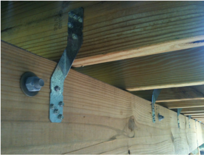
Attach strong ties or clips to solidly connect any beams to the rafters or joists.
