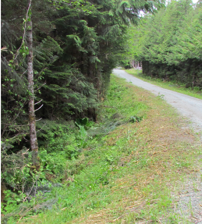
Periodic brush cutting and grading maintains Forest Service road access.
