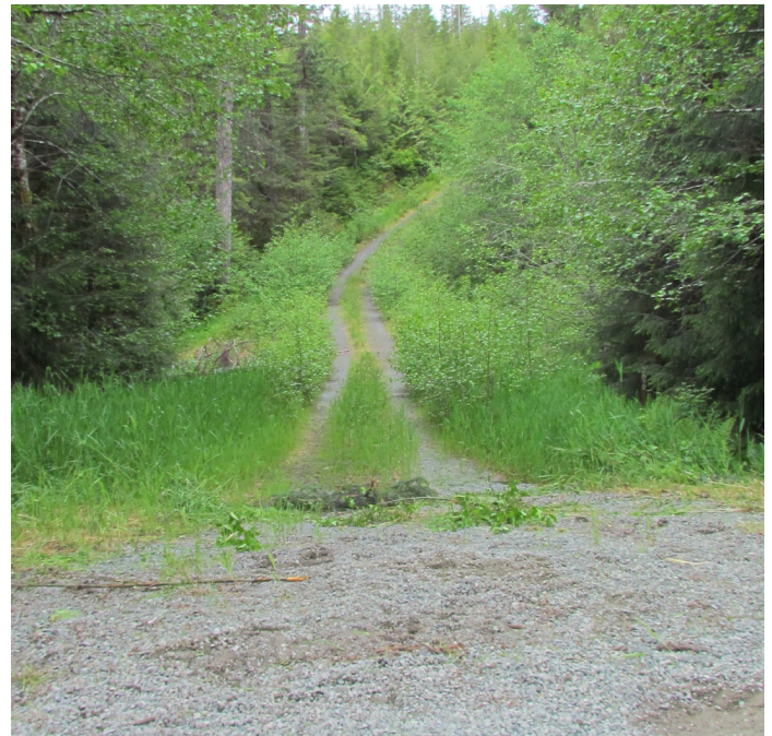
Brush encroachment eventually makes access inoperable.
