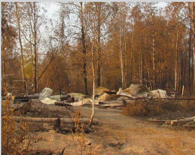
This shows the aftermath of the 2019 McKinley wildfire near Willow, Alaska. Creating defensible space might have helped saved this structure.
