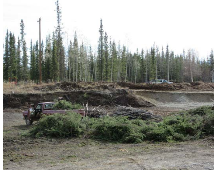
A brush disposal site for people to dispose of brush, thinned and pruned material helps reduce on-site fire danger.
