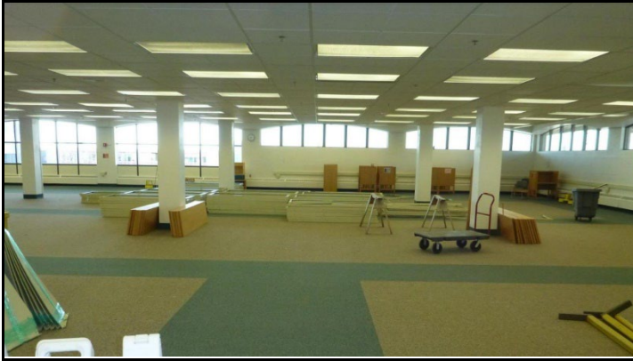
The 6th floor of the library all cleared out and ready for renovation
