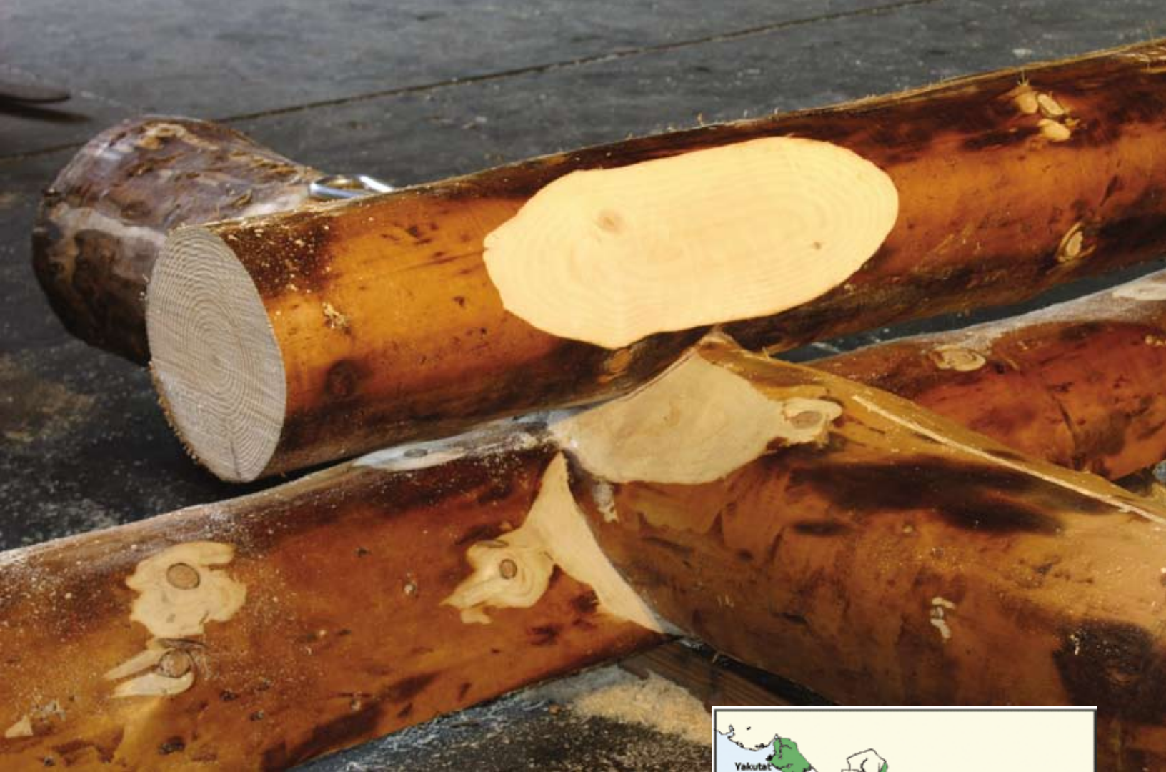
Above: notched logs in the preassembly stage at the hangar on the Sitka campus.
